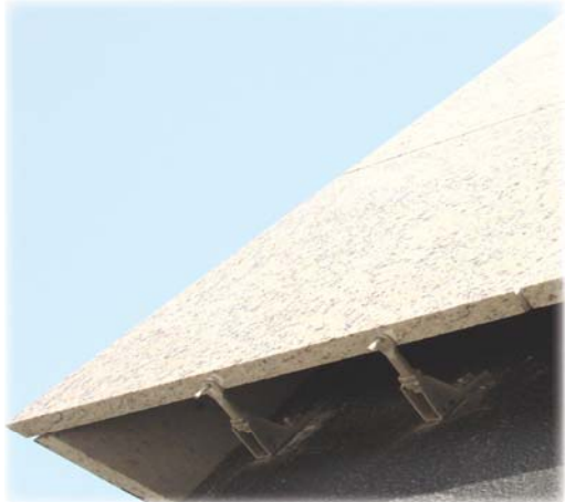
• AX01 Anchors used to install slabs on to blockwork walls.
