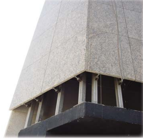
• Special HMPA sub channel construction.
