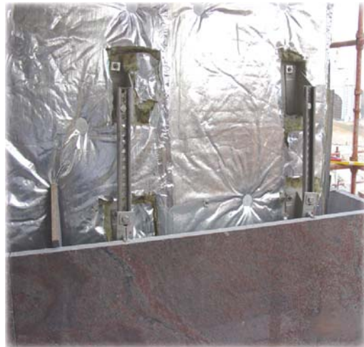
• HMPC-HC1 system used to install slabs onto isolated walls.
