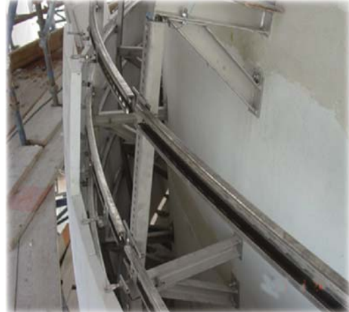
• Special HMPA sub channel construction.
