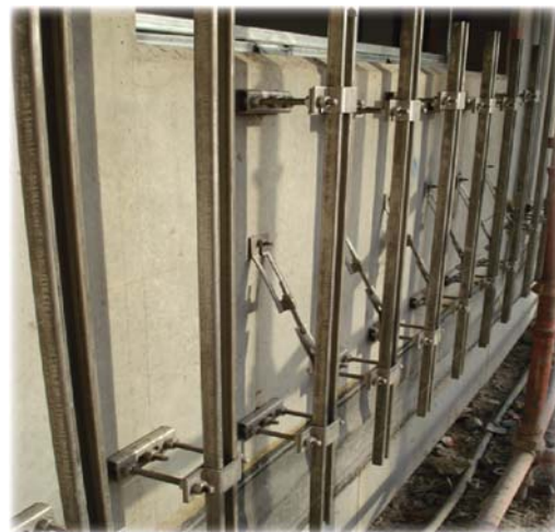
• ATS sub channel system to install slabs below windows.
